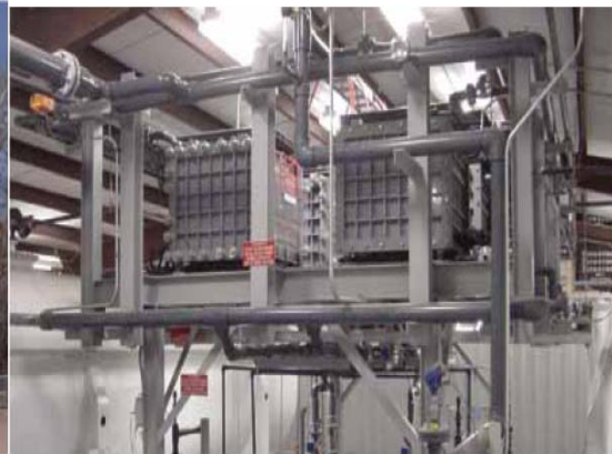
⌘ Exterior and interior views of the 2MWh VRB system at Castle Valley, UT.
