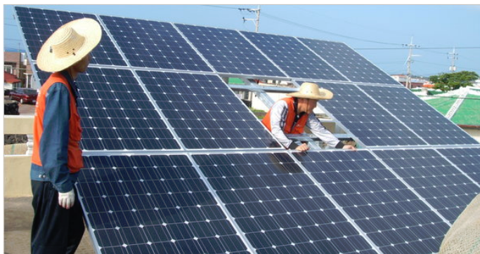
Workers install a solar panel on a household within the Jeju Smart Grid project site. More than 2,000 homes along Jeju's northeastern coast have been connected to the test grid.
